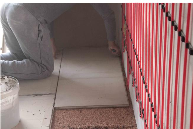
With cement bonded particle boards BetonWood TG with a thickness of 20 mm, excellent thermal insulation can be achieved, as well as a high noise reduction, considering that the thicknesses do not involve problems in terms of weight on the underlying structure.
