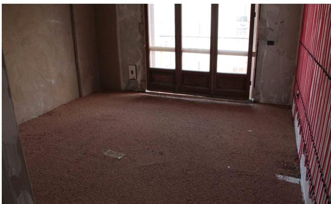
In the case of a totally floating structure on granulated blond cork (as we can see in the figure) we recommend to install cement bonded particle boards with tongue&groove edges BetonWood TG laid by staggering the joints and screwed on each other, with offset arrangement.
