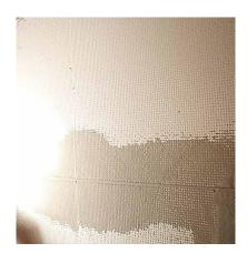
Starting from top to bottom, the high-density BetonNet Glass 360 glass fiber mesh is unrolled (360  $gr/m^2$ ); the overlap of the nets must be about 10 cm.
